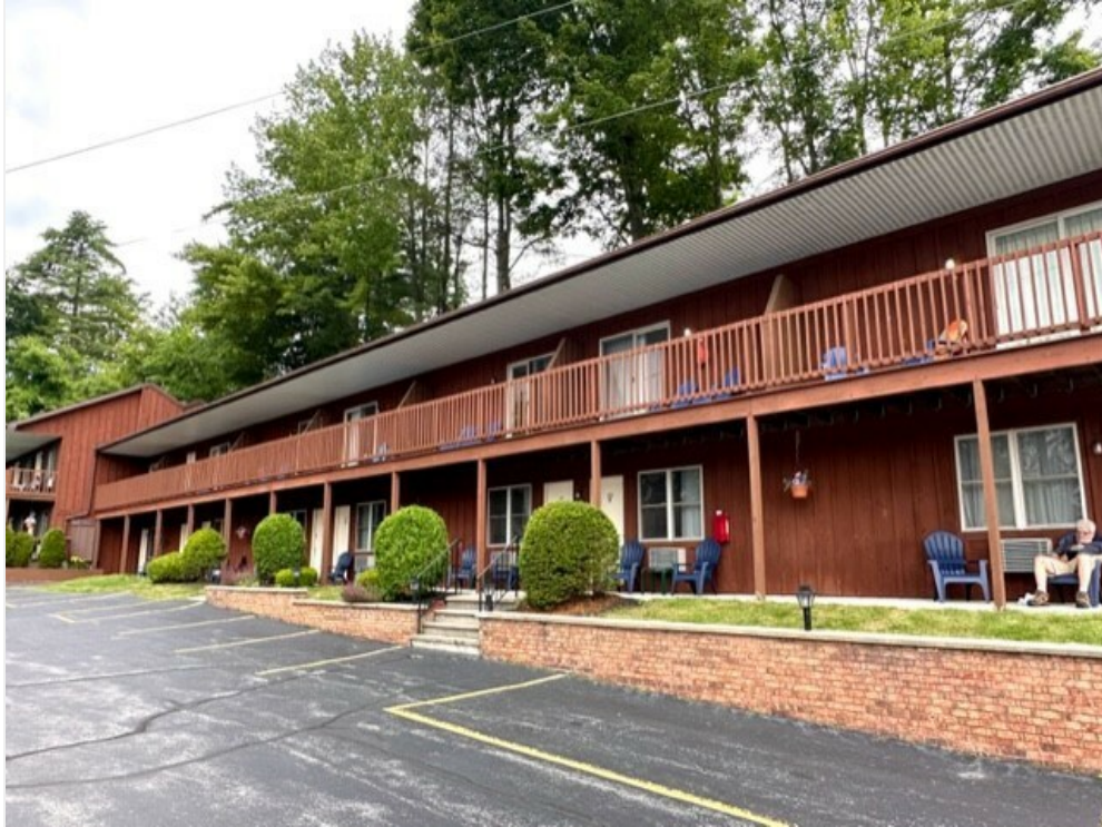
Exterior Rooms Building
